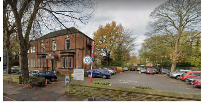
The Bridge Club
