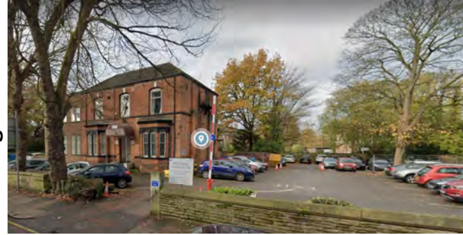
The Bridge Club
