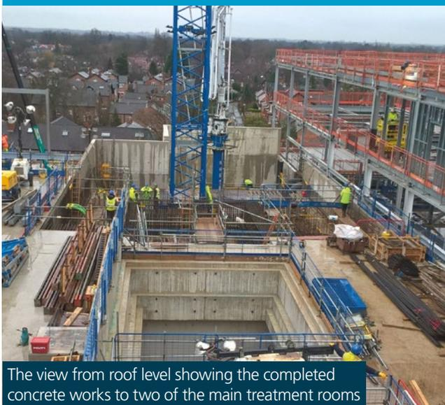
The view from roof level showing the completed concrete works to two of the main treatment rooms
