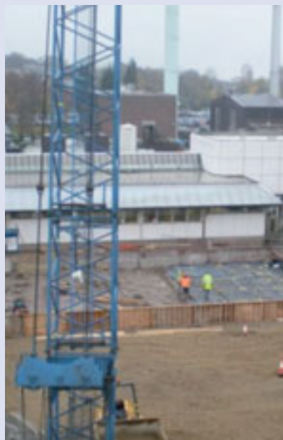
▲ Under construction: Our new radiotherapy centre in Oldham.
